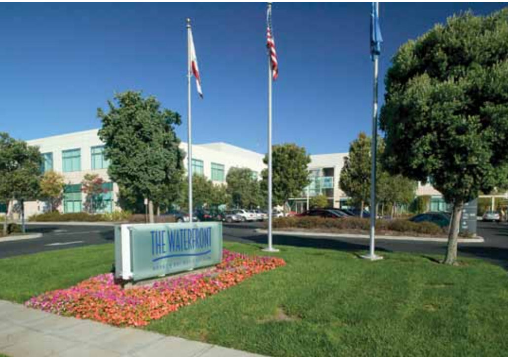
The Waterfront at Harbor Bay, Alameda, CA
